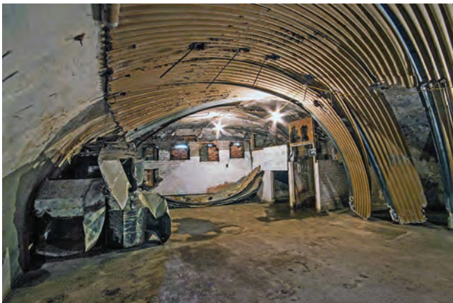
BBC plant room looking towards the external wall
